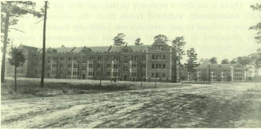
The University of Florida in 1906. Thomas Hall (foreground) and Buckman Hall were the only buildings available in Gainesville during Sledd's presidency. Both were built with the $70,000 donation by the City of Gainesville to acquire the university. Image courtesy of the University of Florida Department of Special and Area Studies Collections.
