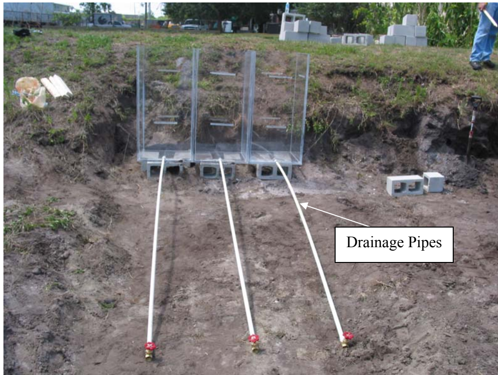
Figure 9 – Chambers before backfill
