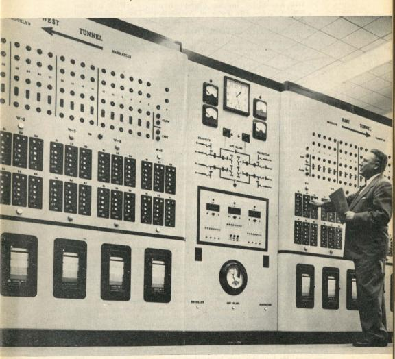
Control brain of the new Brooklyn-Battery Tunnel's electric system. Permits control of ventilation according to carbon monoxide concentration.
