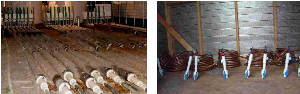
Figure 5-1 Pilot Distribution Systems and Corrosion Loops
