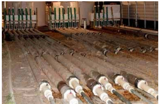
Figure 3-2 Influent Standpipes, Inhibitor Tanks and Pipes System
