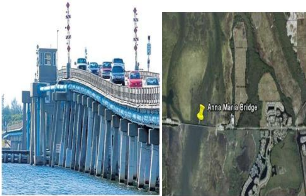
Figure 20: Left: Existing Anna Marie Island Bridge. Right: View of Anna Marie Island in Tampa Bay and Study Bridge Location (Mara & King, 2008)
