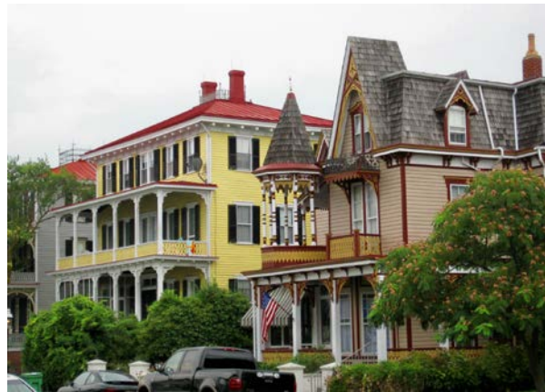
Figure 6: Surviving Cape May Cottages
