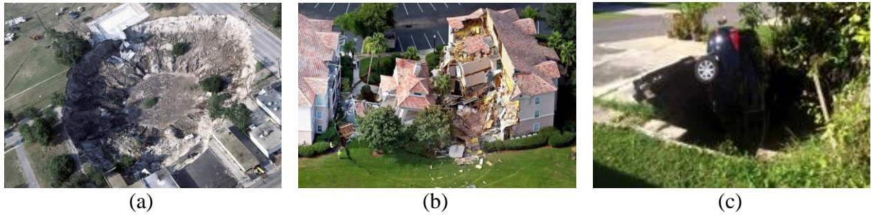
Figure 2-1. Photos of cover-collapse sinkholes in Florida: (a) Winter Park, FL (May, 1981), (b) Orlando, FL (August, 2013), and (c) Pasco County, FL (November, 2014).
