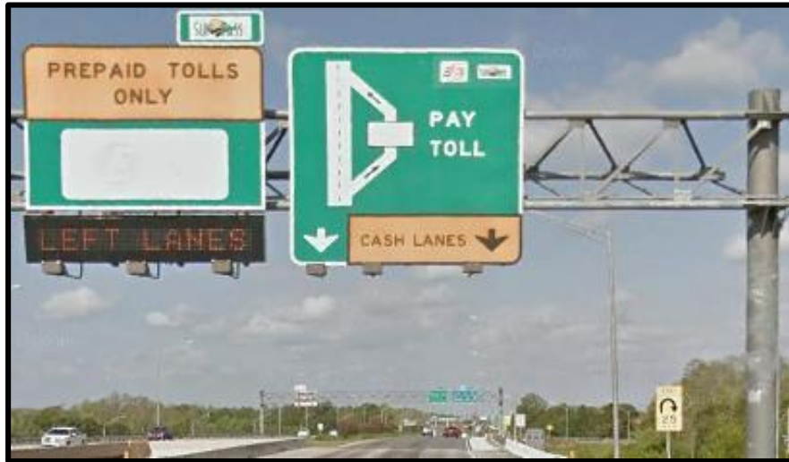
Figure 34. Overhead Sign (Source: Google Earth)
