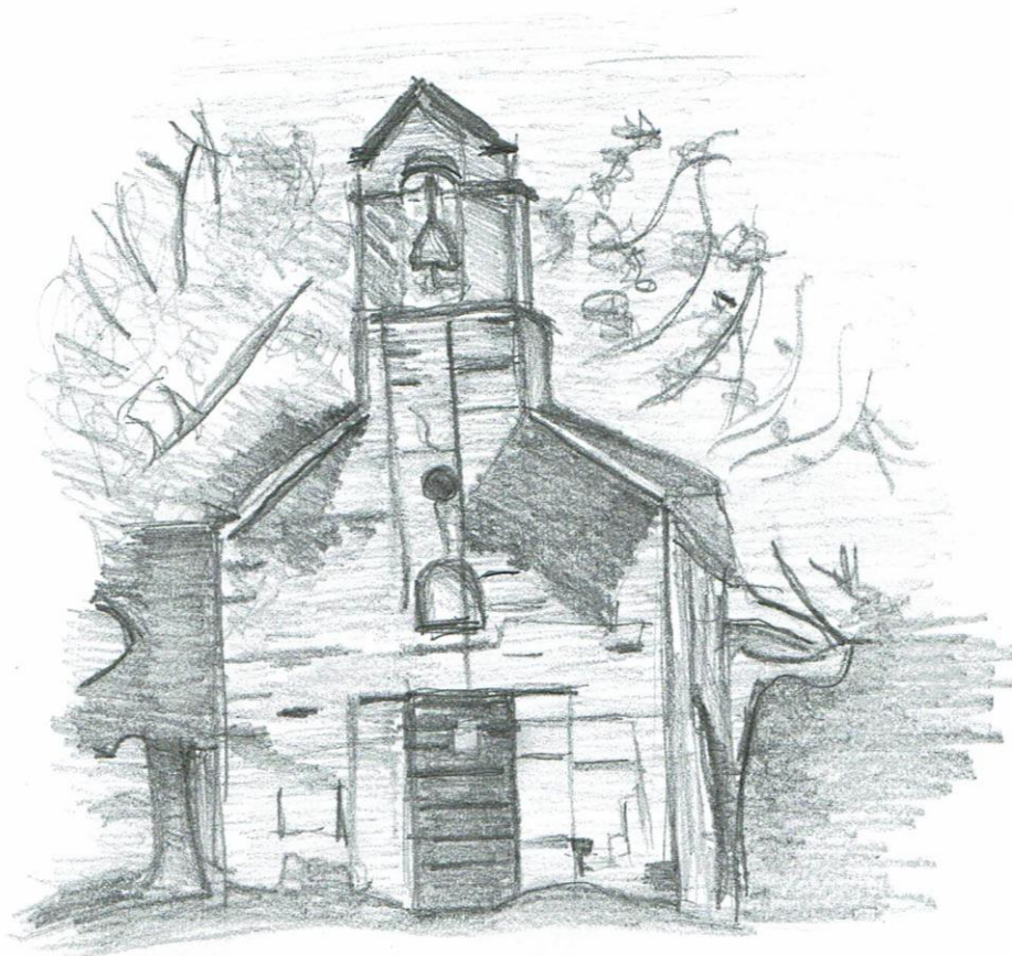
Figure 4 Church of Saint Nicholas at Mistihalj, redrawn after the photograph (Bešlagić, 1962).
