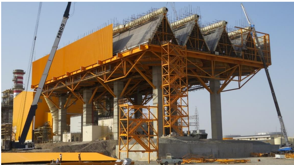
Figure 2.13: Construction of a combined-cycle power plant air-cooled condenser
