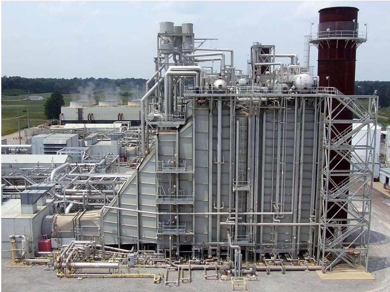
Figure 2.6: Triple-pressure heat recovery steam generator
