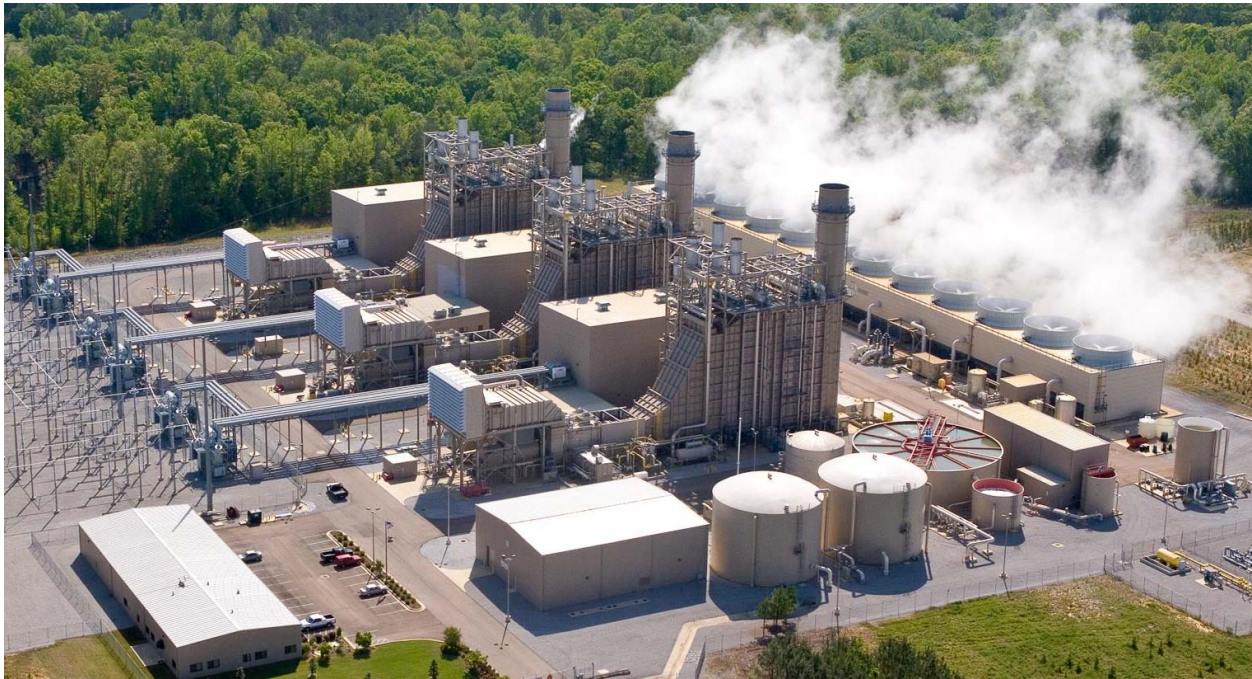
Figure 2.2: TVA Caledonia Combined-Cycle Plant, Mississippi
